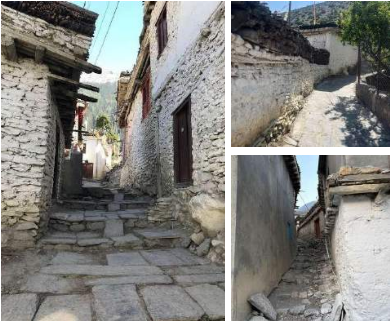
Traditional Pedestrian Street Network of Thini Village Showing Narrow Stone-Paved Lanes and Vernacular Residential Architecture.
