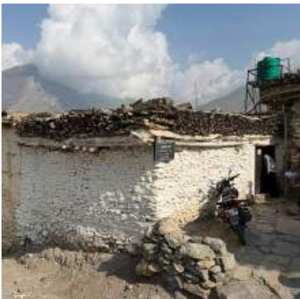
Stone Masonry on Mud Mortar
