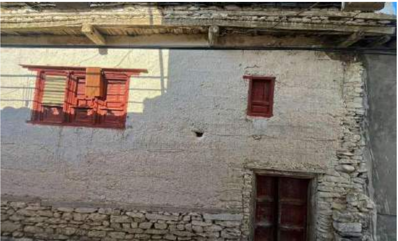
Main entrance to the livestock goth in a well-preserved 200-year-old Thini house.
