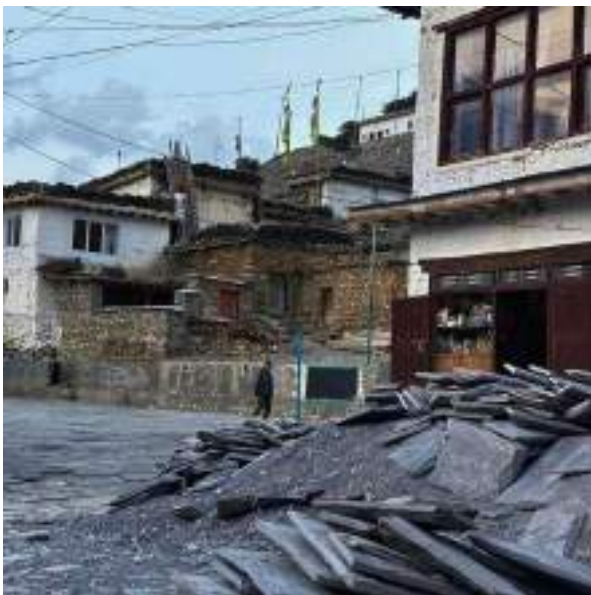
Stone Masonry and Rammed Earth
