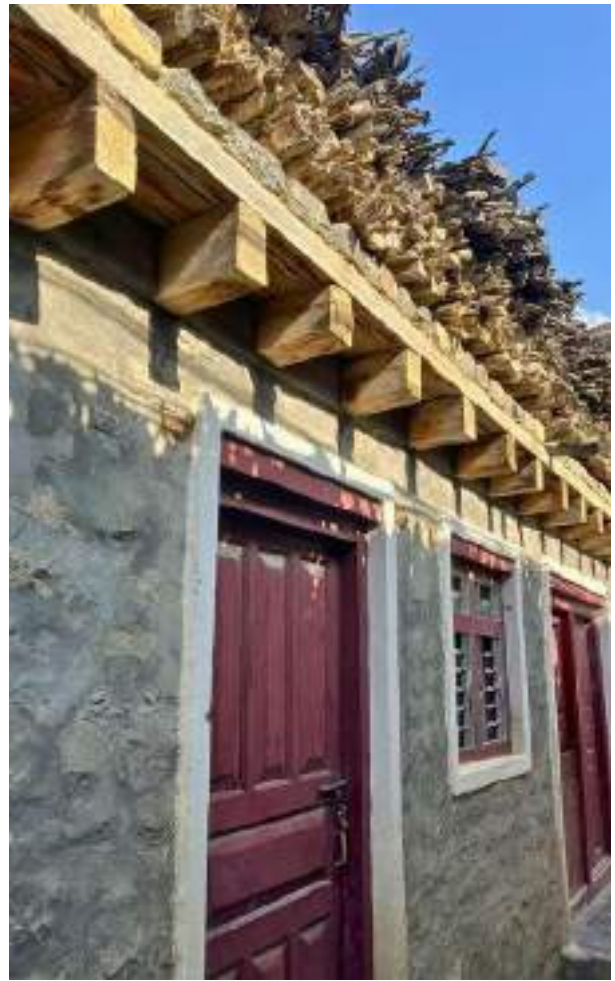
Traditional stone façade with timber roof overhang
