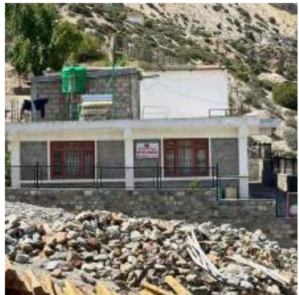
RCC Framed with Stone Masonry
