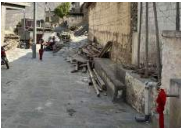
Community Water Tap
